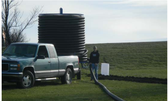
Nick Donahue helps drag drain tile through trench .
