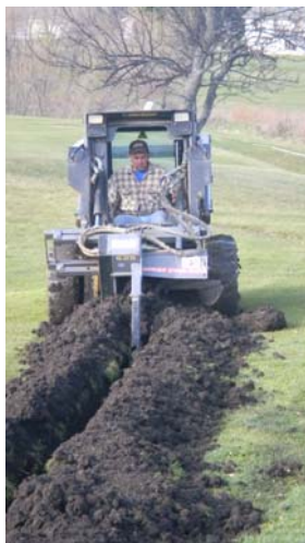
Tom Lundberg trenching in drain tile.
