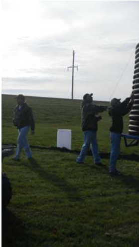
Mike Donahue, Larry Molitor and Nick Donahue unloading drain tile
